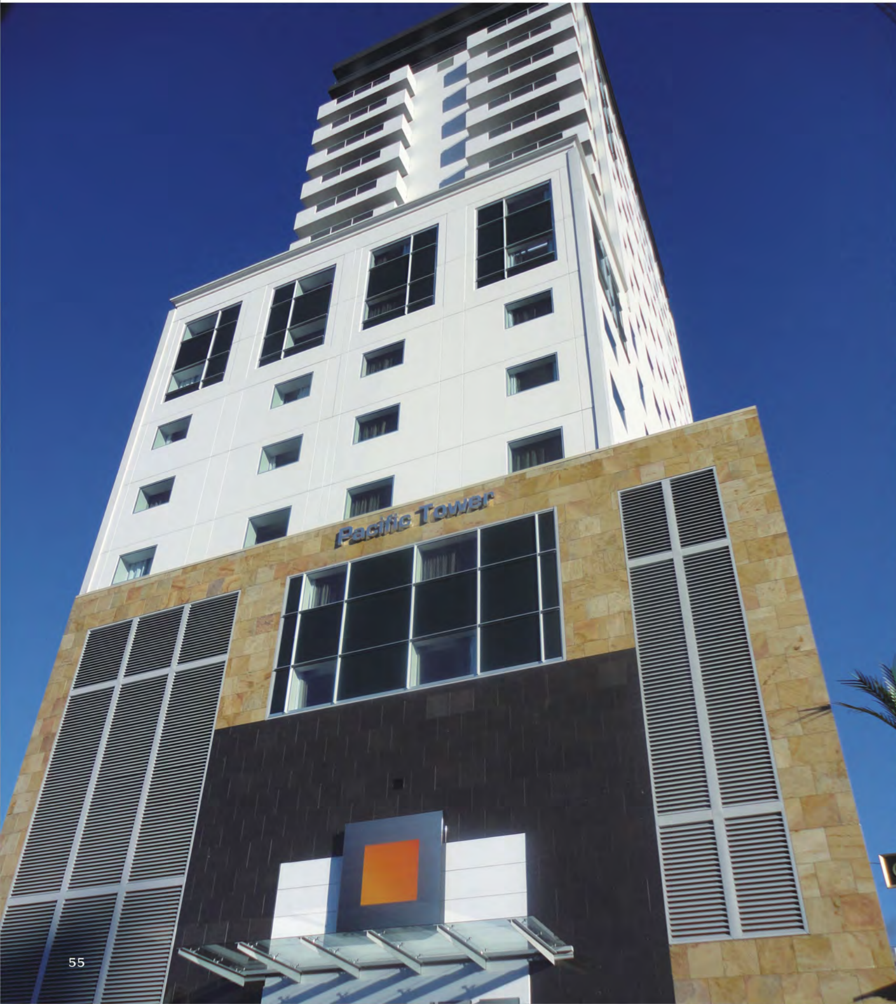
Pacific Tower, Christchurch, New Zealand
