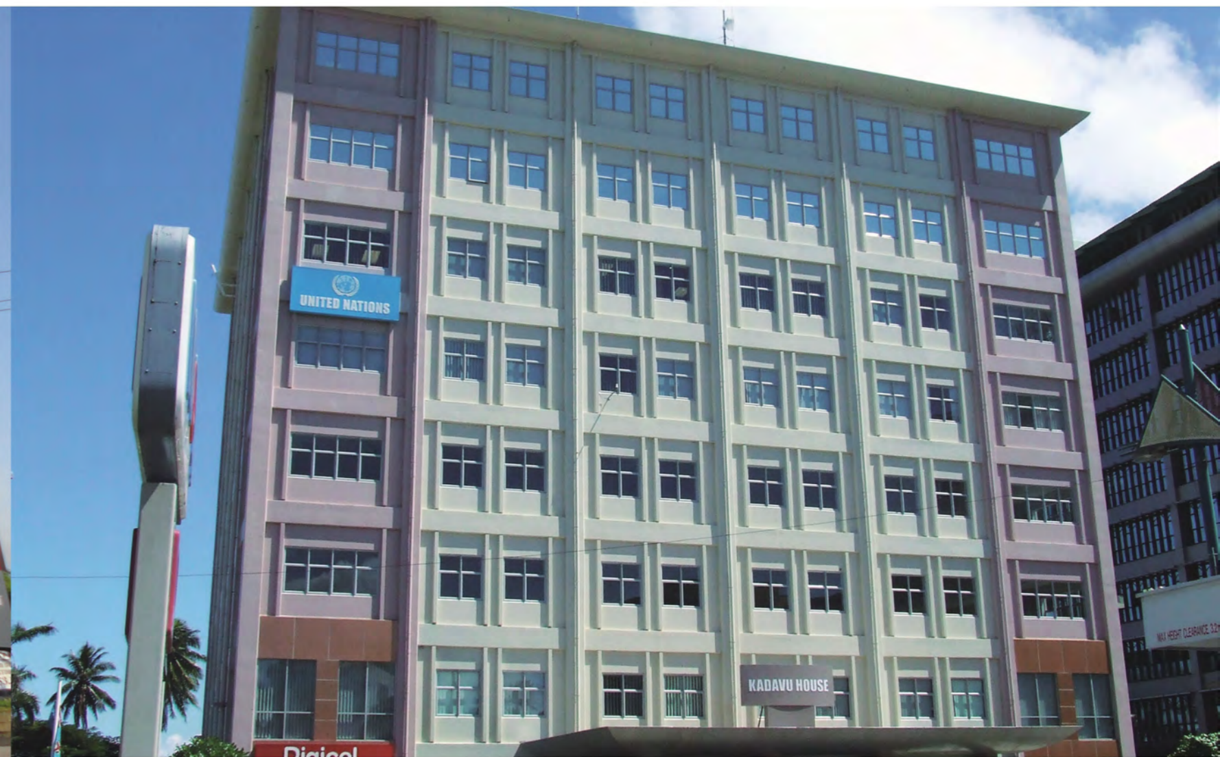
Kadavu House United Nations Office, Suva, Fiji
